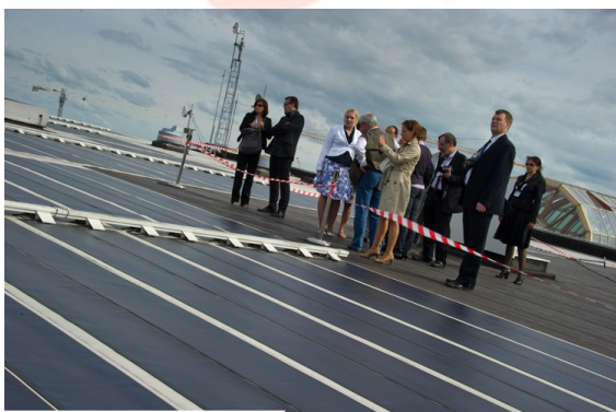
Seminar participants visited the rooftop solar installation at Flanders Expo.
