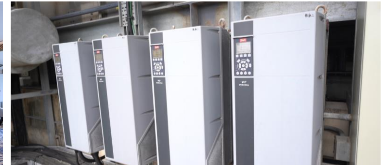
Replacement of Water-cooled chillers reducing >3840tCO2e = planting of >167,000trees
